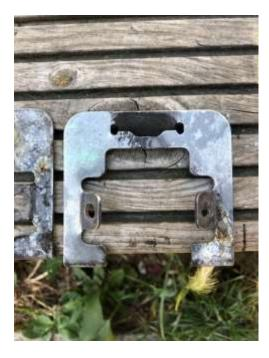
Plate Installed with A4 Marine grade Stainless Bolts, these will get a tiny bit of Locktite on final assembly
